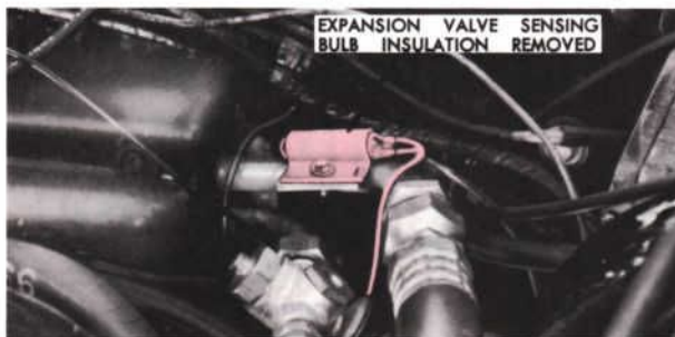
Figure 16—Checking Expansion Valve Bulb Contact
